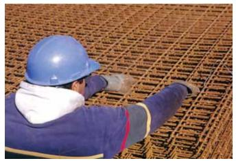
applicable industry standards. Inspect reinforcing cages for size, spacing, proper bends and length. Secure the reinforcing cage in the form so that shifting will not occur during casting. Use only chairs, wheels and spacers made of noncorrosive materials.
