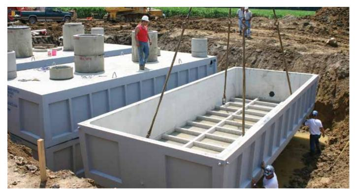
Baffles or tees are permitted to be precast monolithically with the tank. If baffles, tees or outlet filters are added, they shall be made of non-corrosive materials and be permanently connected with noncorrosive fasteners to either the inside of the tank or the outlet pipe.
