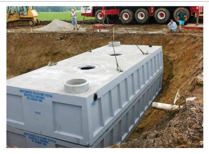
Precast Concrete Water and Wastewater Structures;" and C913, "Standard Specification for Precast Reinforced Water and Wastewater Structures."
